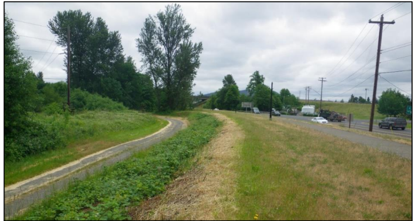
Figure 2: Typical 42 nd Street Levee section north of Highway 126 (42 nd Street at right).
