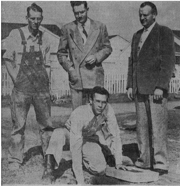
JAY HICKS, JR., superintendent of the new Rainbow Water District north of Springfield, turns on a meter for the new system which is going into service this week. Watching him are Paul A. Braun, foreman for Inter-City Sand and Gravel, which did the job; Albert A. Brown, secretary of the board, and Adrian Vaaler, engineer. The new system, which will serve 300 users when it is hooked up, will depend on more than 40,000 feet of pipe. Water will be purchased from the Eugene Water and Electric Board.
