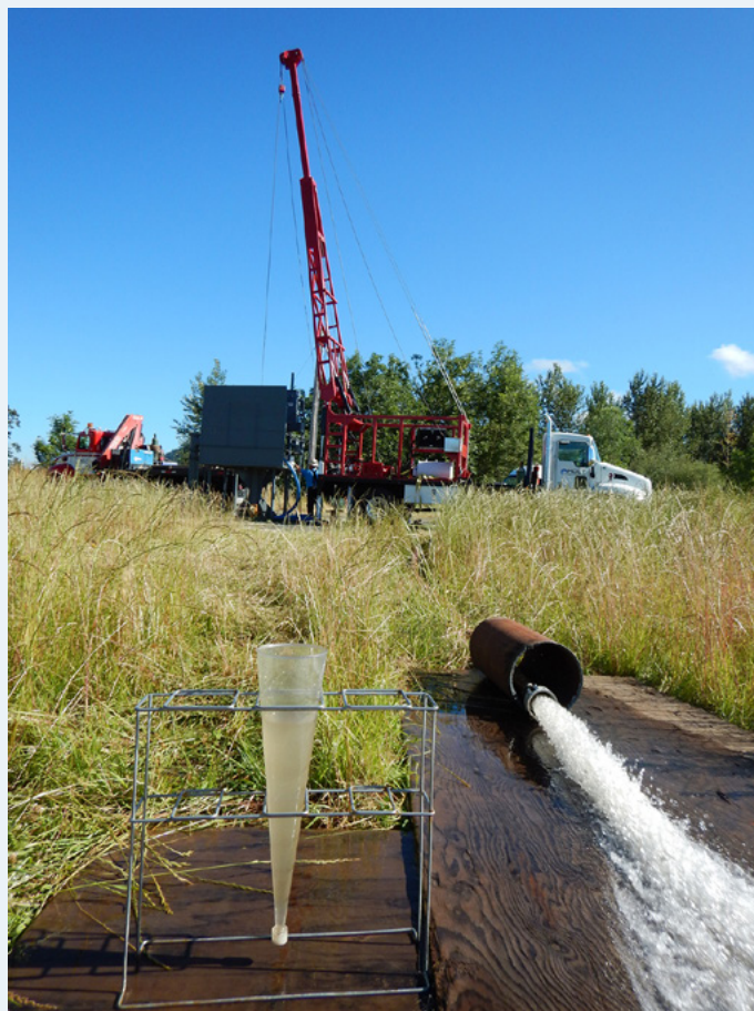
Well rehabilitation to improve productivity
